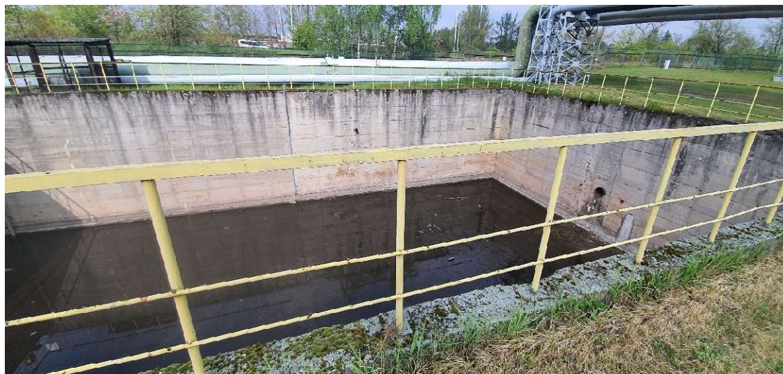
Figure 12 Water reservoir in the vicinity of the investment project
